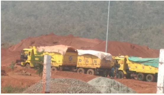
Figure 26 Laterite being dumped at the bottom of the hill
